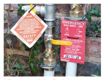
A. Emergency control valve - Closed valve
