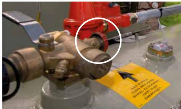
B. Above-ground tank gas isolation valve - Red hand-wheel circled above
